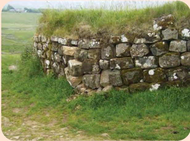
Clayton Wall at Steel Rigg in danger of collapse © HWHL
