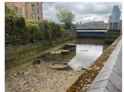
Progress photo at Swan Draw Dock
