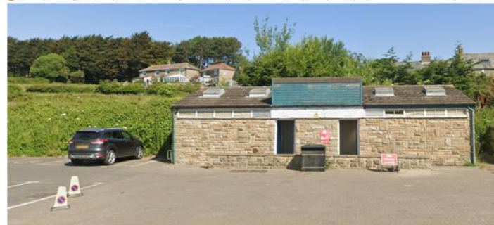
Figure 82. Station car park has 2 small accessible bays and a toilet block in need of update.
