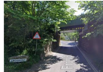
Figure 71. Narrow road, no footpath.
