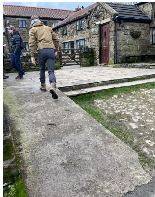
Figure 61. Ramp access from car park to single step main entrance. Image © Natural England.
