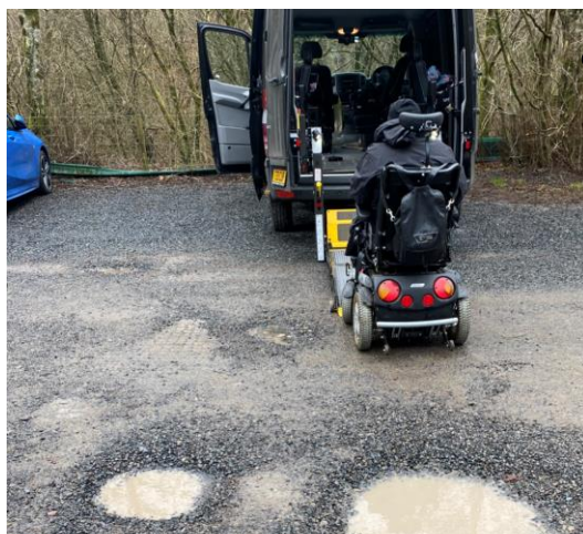
Figure 29. Repair potholes, provide firm surface for Blue Badge parking. Image © Natural England.
