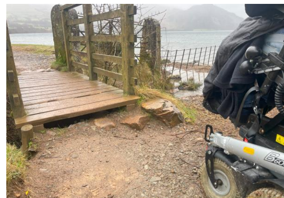
Figure 123. Route 23 - Inaccessible Bridge at the foot of 1:8 path. Uneven, severe camber. Image ©Natural England.
